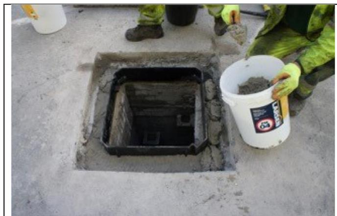
10.3 All old bedding mortar is removed, and the supporting structure is cut back or loose bricks are removed, until a sound base is achieved.
