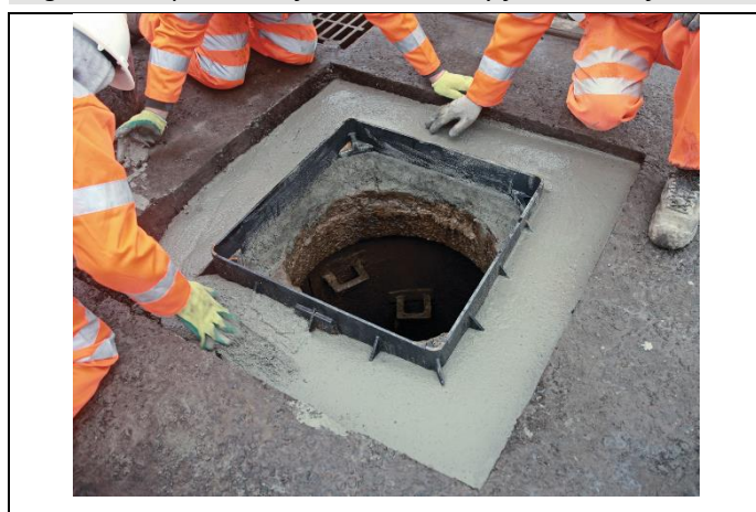
Figure 1 Preparation of substrate ready for the backfill
