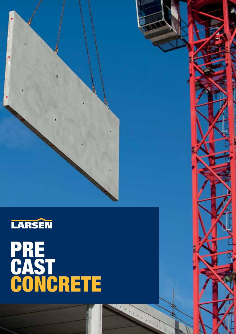
Precast concrete applications push the boundaries of concrete both in terms of performance and quality of finish. Much greater control is afforded to the producer by forming concrete off-site and this control creates cost benefits. The effective use of admixtures can create high strength fluid concretes which allow the production of thin, highly reinforced structural elements which reduce the overall building cost.
